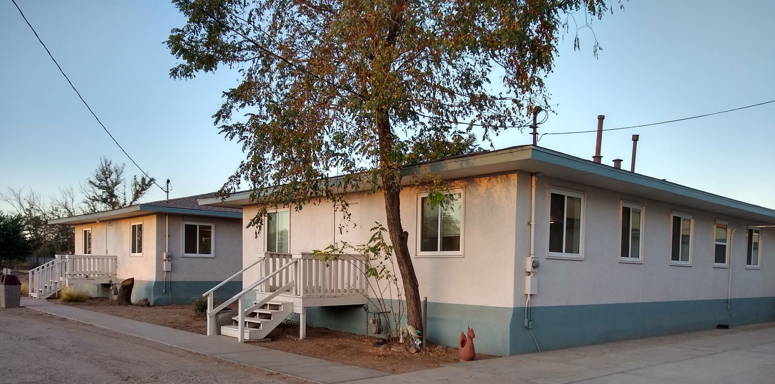
New Look of Back of Barracks
